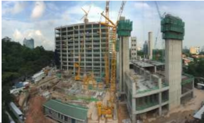
Phase 2: Superstructure works in progress
