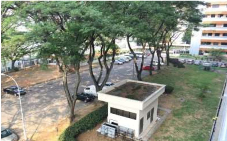
Development of Hi-Tech Building at existing car park
